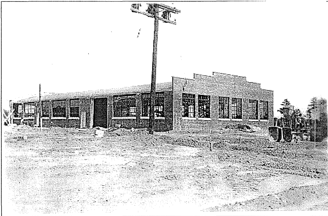
Figure 15 - Building 446 (Repair Shop), 1939
